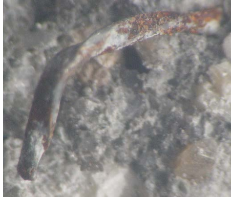
Figure 2.18 Pullout failure despite the onset of corrosion; fiber observed in sample CI1 observed under the stereographic microscope Photograph by Dietrich Vogel copyright 2016 by Dietrich Vogel
